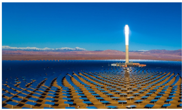
Concentrated Solar Tower
